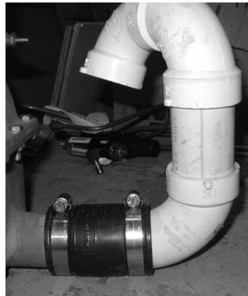
Photo 6 – No-hub connector connects a fabricated p-trap to the ejection chamber.
