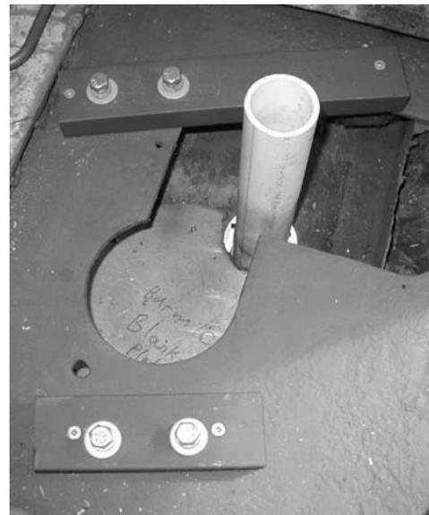
Photo 5 – Inverted channel in floor provides a sturdy mount for the toilet.
