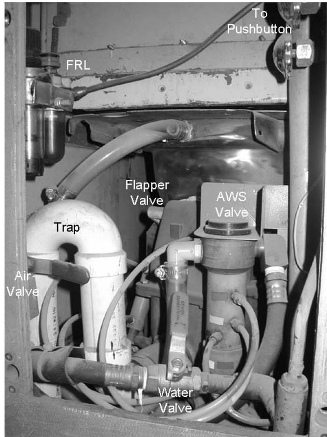
Photo 8 – System components installed behind a roomette toilet.
